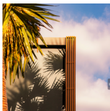
THE VICTORY BY ANDAMAN ASSET SOLUTION
